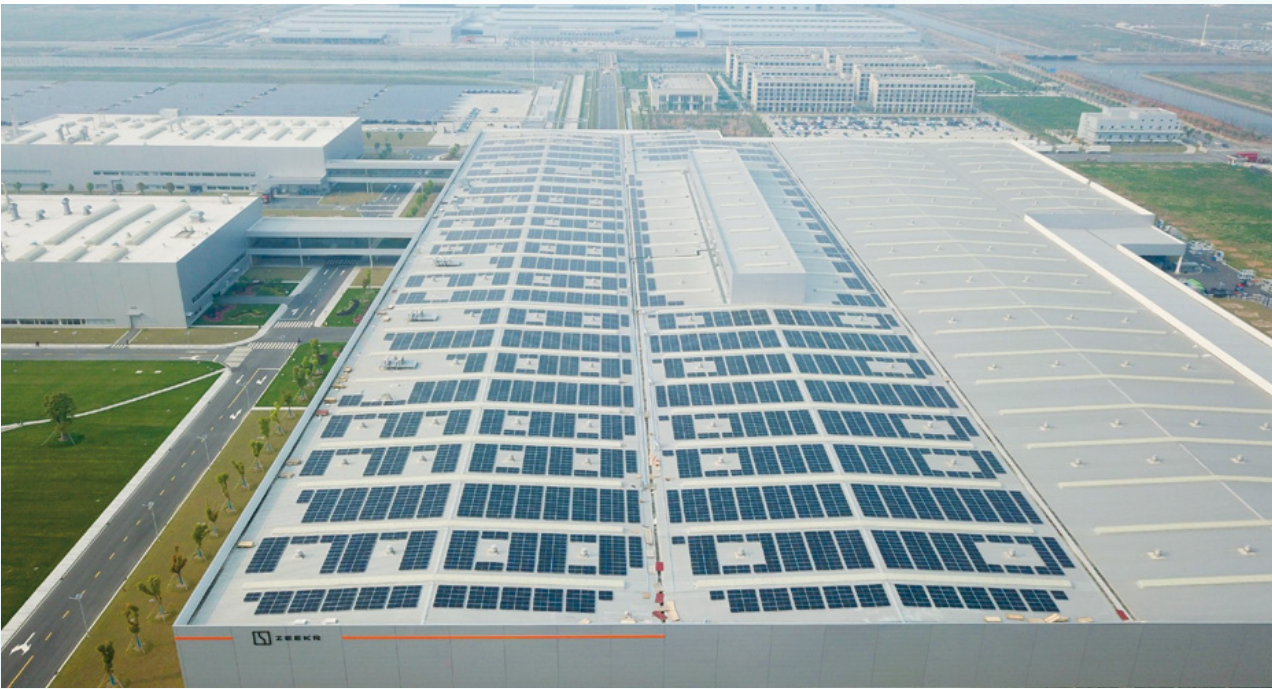
The installed capacity of rooftop photovoltaics in ZEEKR's factory reached 29.46MW. Besides PV systems, ZEEKR's factory will also fully implement green-electricity-certified procurement starting in 2022
